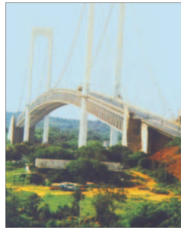
With its program of public works Bolívar is building links to the more remote parts of the region.
