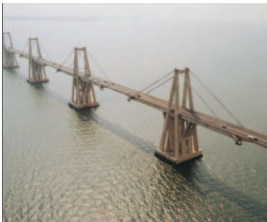
Building bridges. Zulia is investing heavily in improved infrastructure.
