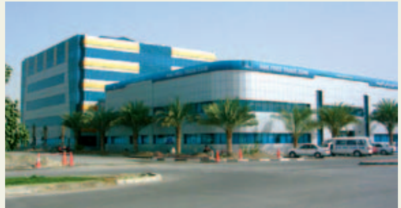
RAK FTZ covers the emirate's access points, including the airport and the Saqr Port.
