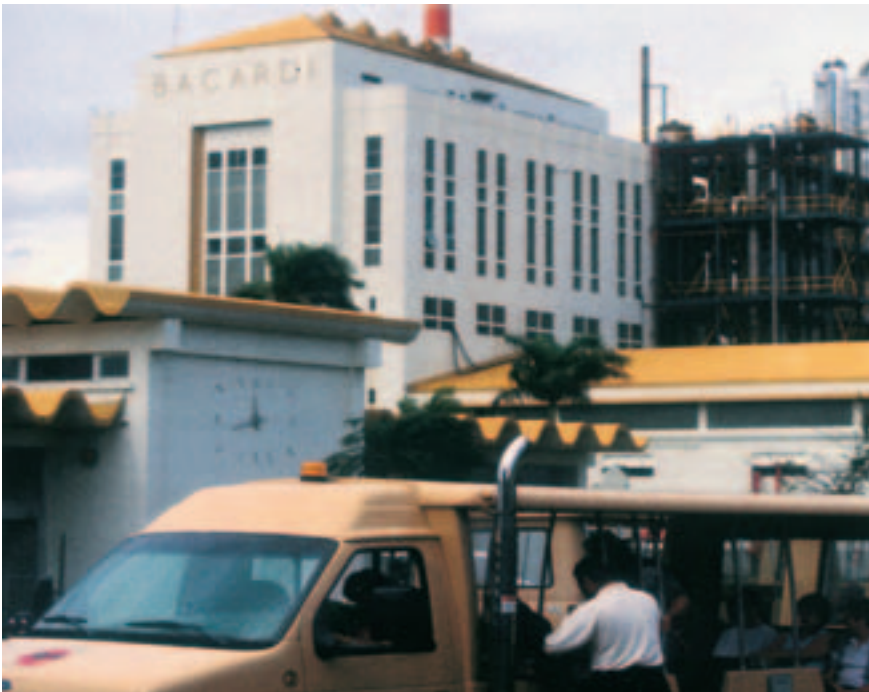
THE GOVERNMENT would like to develop high-tech industries and spur manufacturing
