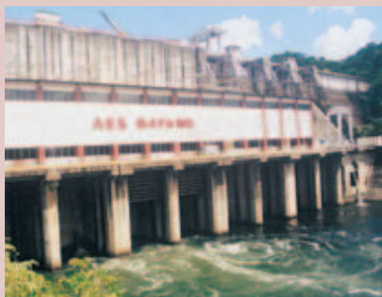
POWER TO THE PEOPLE: AES Panama's Bayano hydroelectric plant.
