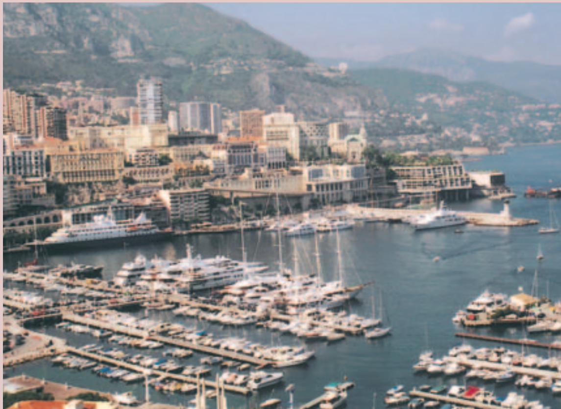
PORT PLAN The extension and refurbishment of Port Hercule, currently under way, will boost the luxury yachting sector and increase cruise tourism
