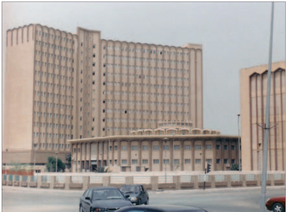
The headquarters of the General Post and Telecommunication Company, which is responsible for both fixed-line and cellular phone networks.
