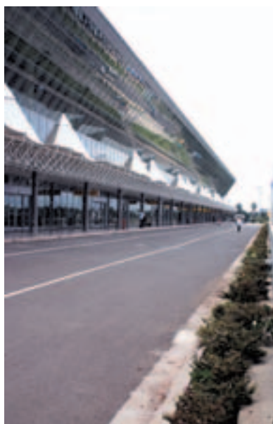
The upgrading of Ethiopia's Addis Ababa Bole International Airport is backed by multi-million dollar loans from the fund.
