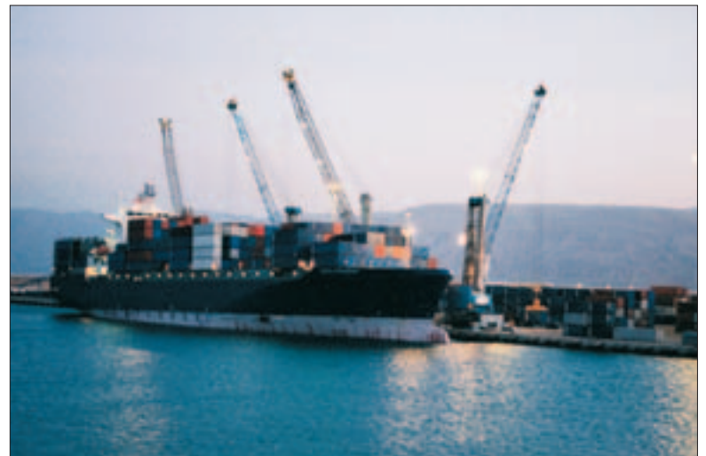
State-of-the-art equipment has turned Sokhna into one of the world's most sophisticated ports
