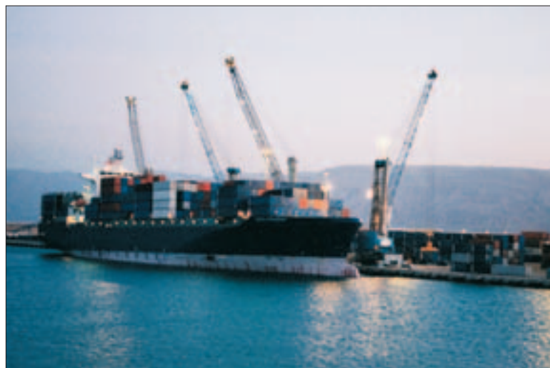
State-of-the-art equipment has turned Sokhna into one of the world's most sophisticated ports
