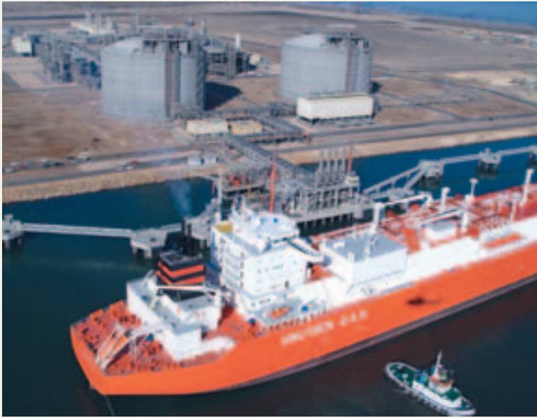
The Mubarak liquefaction and export complex in Damietta.
