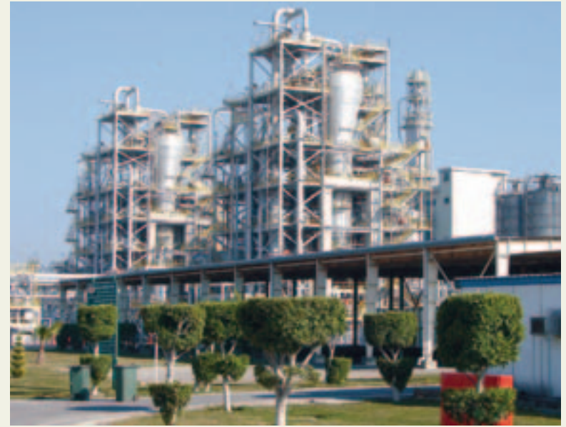
Sidpec's expansion plans include opening two new plants for ethylene and polyethylene.
